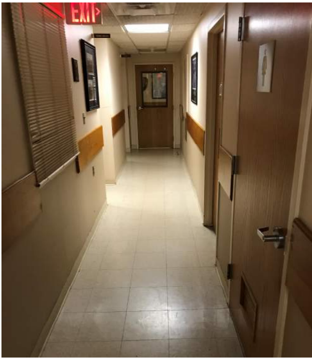
Narrow Corridors with Out-Swinging Doors
