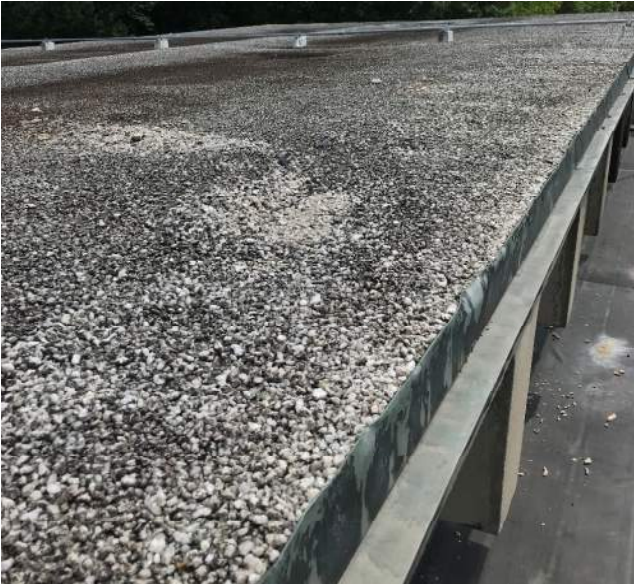
Existing Built-Up Roofing
