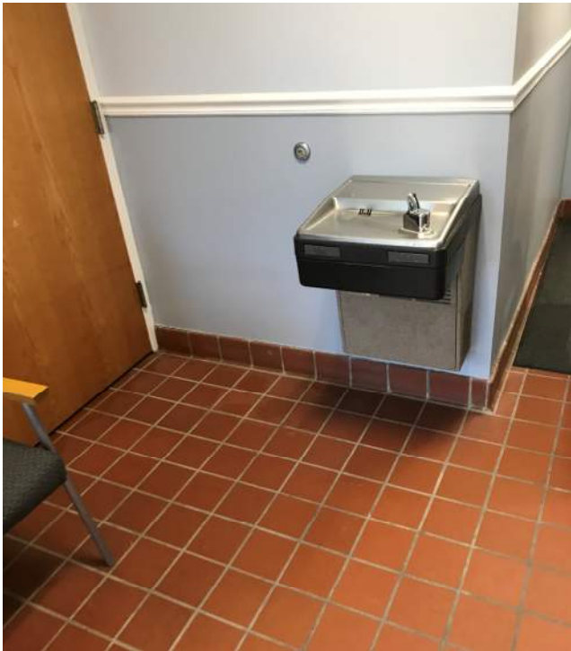
Non-ADA Accessible Water Fountain
