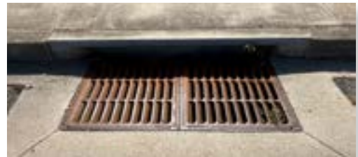
Storm drain inlet grate on Gateway Drive
