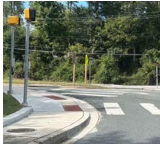
Improvements at John Carroll School intersection on MD Route 22
