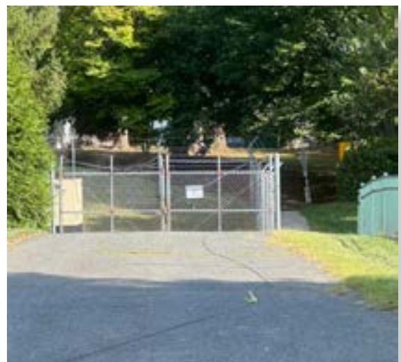
Missing sidewalk between Roland Place and Dallam Avenue
