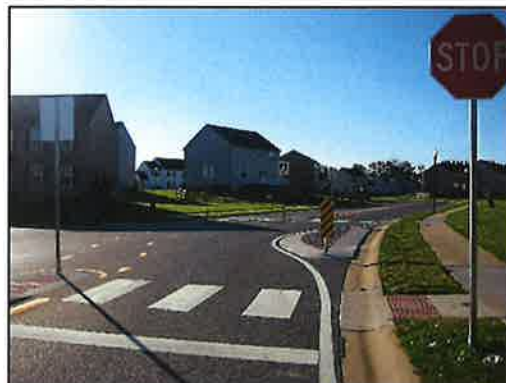
(Source: Delaware DOT)
