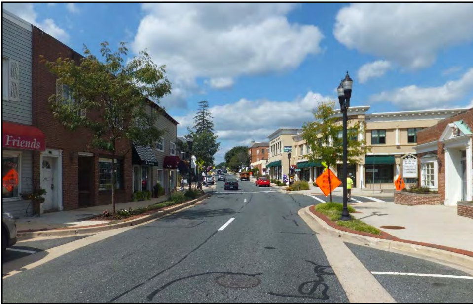
Figure 4. Main Street Approach to Lee Street
