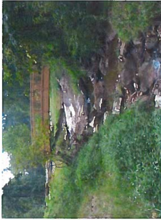
(b) Same reaches six months after restoration with log/boulder step-pools
