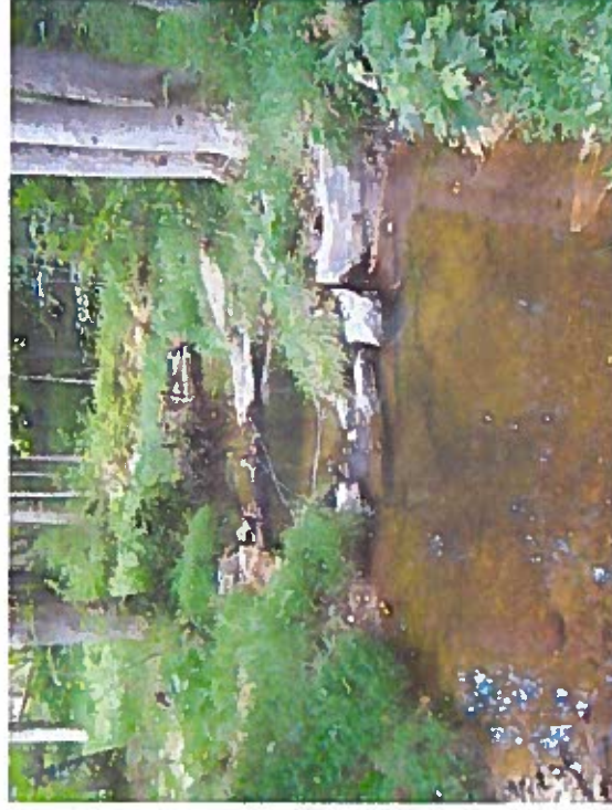
(b) Same reaches six months after restoration with log/boulder step-pools
