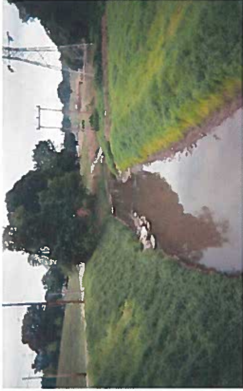
(b) Same reach four months after restoration with toe benches and soil fabric lifts. Note channel has been shifted away from failing slope and narrowed.
