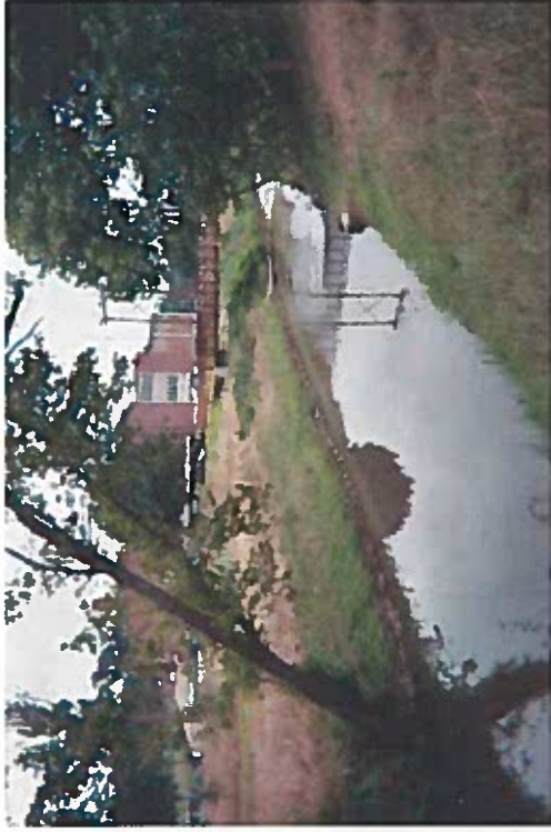
(b) Four months after restoration with toe benches. Note channel has been narrowed significantly.
